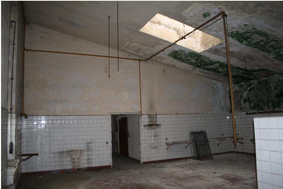
Figure 15 Colonia Elioterapica in 2011: view of the abandoned kitchen.
