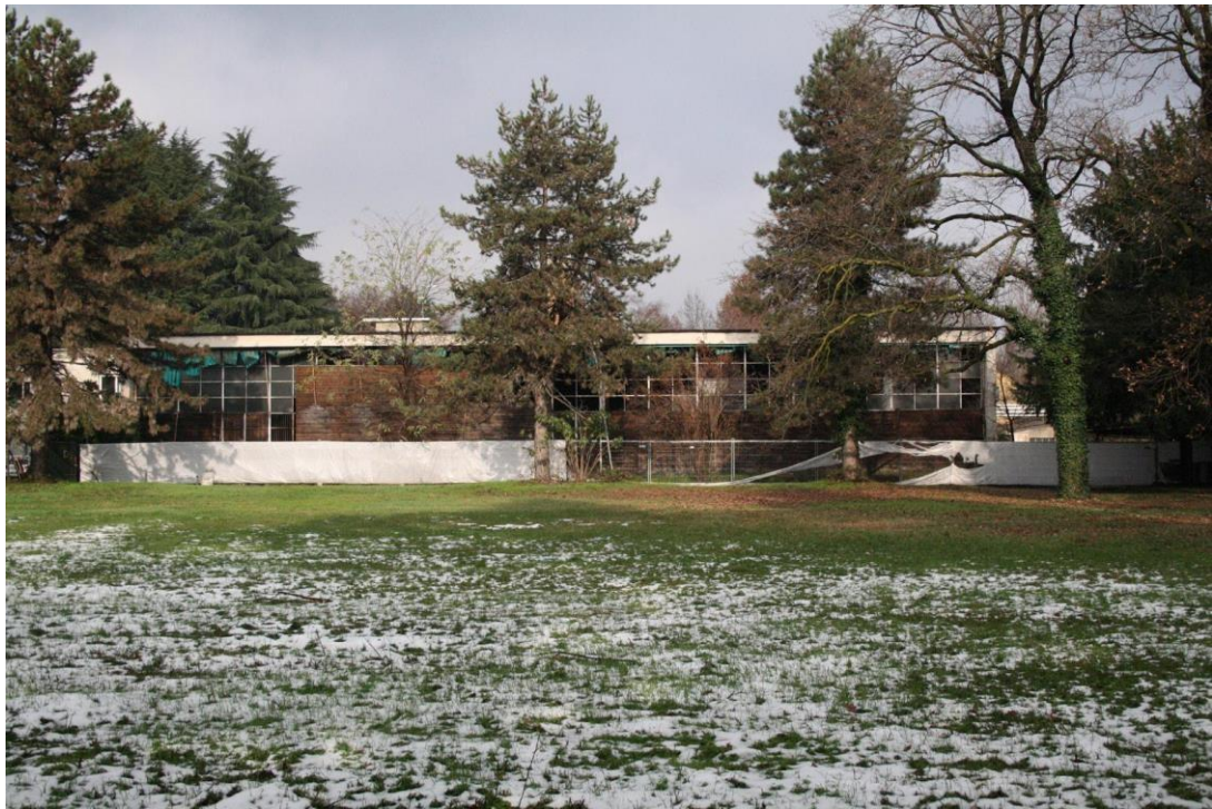
Figure 13 Colonia Elioterapica in 2011: view of the continuous facade.
