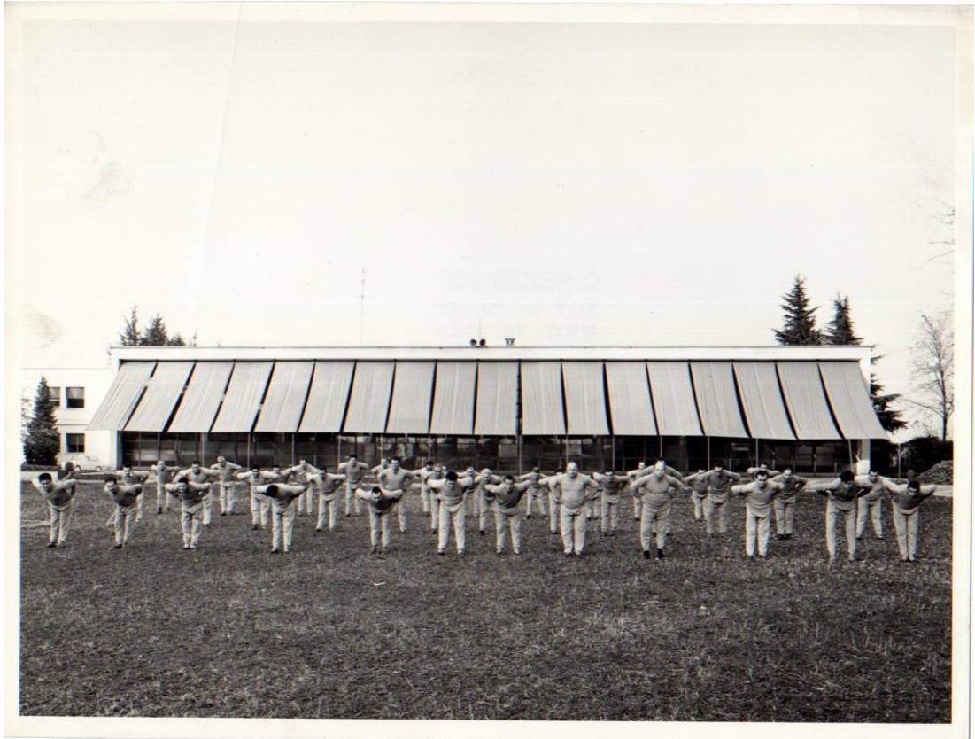
Figure 8 Colonia Elioterapica in 1955: view of the continuous facade.
